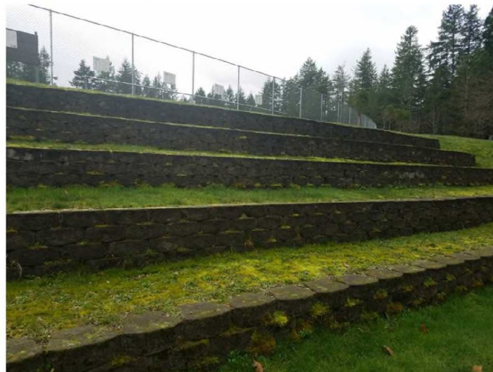
Figure 1.a-4 Grass Terracing With Block Walls
